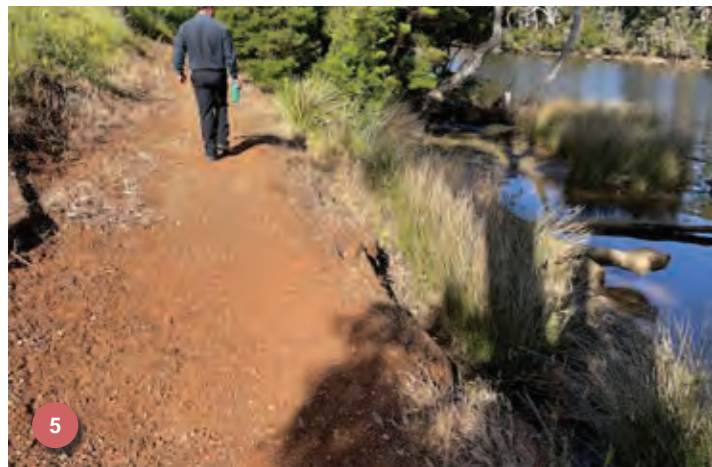
Image: Red soil eroding on the north bank near Cape Bridge
