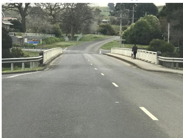
Figure 44 – Saunders St. Southern approach to Table Cape Bridge
