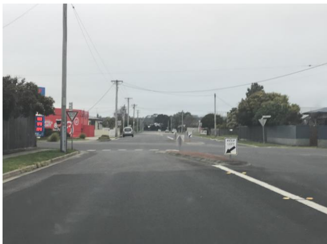
Figure 9 – Austin St. (North) approach to Inglis St.
