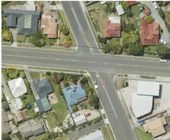
Figure 5– Aerial view of Inglis St. / Austin St. junction
