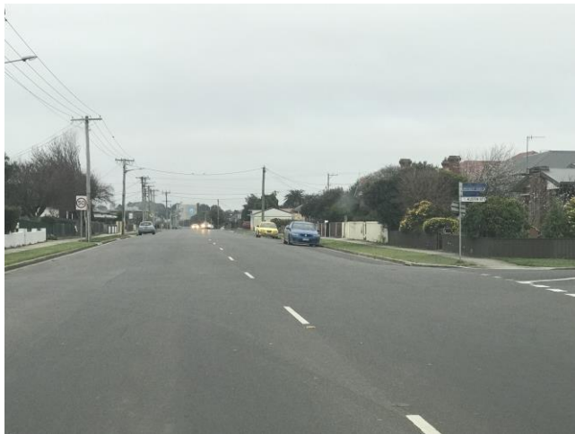
Figure 8 – Inglis Street Eastern approach to Austin St.
