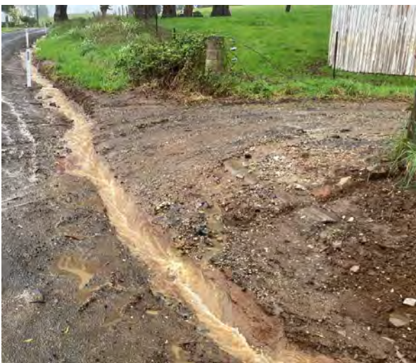
Figure 3: Swale Drain with Scouring Defect
