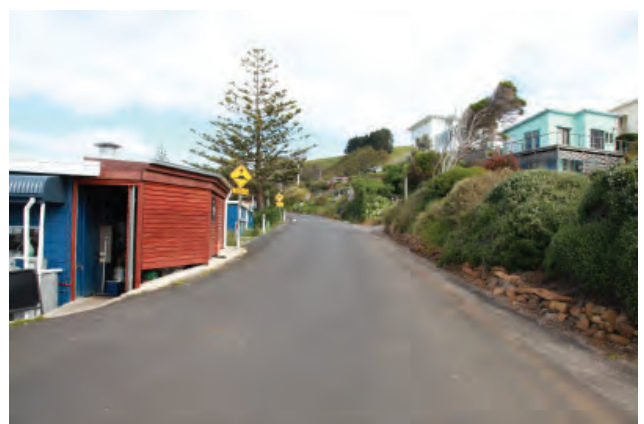
Port Road near the kiosk. The width of the road here often provides challenges during summer months with car parks on the side of the road and patrons lined up at the kiosk.
